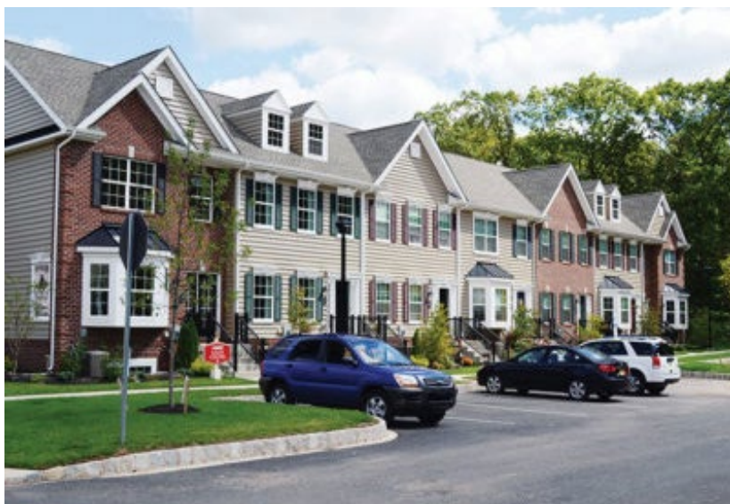
In dense developments with townhomes or condos such as Carriage Hill, community propane systems eliminate the need for on-lot propane storage.
