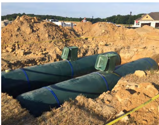
Each home at Bay Bridge Cove has an individually metered propane connection, with lines running to centralized propane storage tanks buried in common space. Homeowners are billed for propane by usage, just as they would be for natural gas service.
